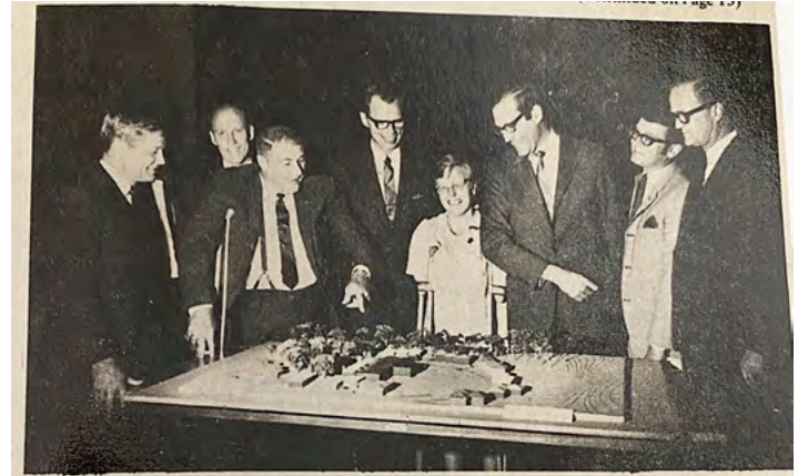
HANDICAP VILLAGE DISCUSSED —Willis Schellberg, architect for Handicap Village was on hand at second annual meeting of the Village corporation Monday night to explain details of construction. Interested persons are (left to right) Dr. Rae Bieber, Peter Murley Severtson, Don Boyer, Bill Otterman, Dr. Anne Carlsen, Schellberg, Wayne Oltrogge and Joseph Skram.
